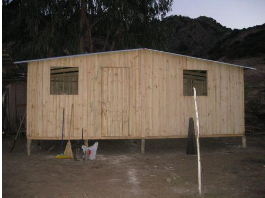
Figure 6. Finished mediagua Photo taken by fellow volunteer, May 16, 2010.
